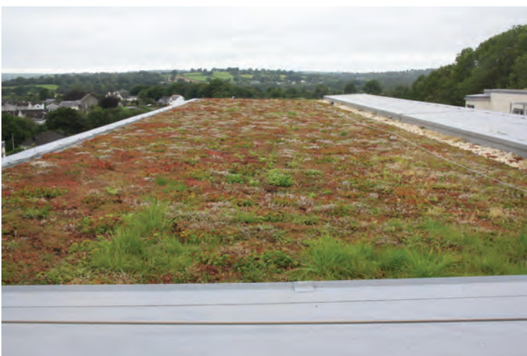
Picture 5.4 Living Roof (Copyright Chris Jones)
